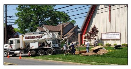
After the concrete had set, the wood had to be removed and a truck poured concrete to fill the hole. After this, a truck was required to move the 500 pound sign onto the concrete base. This was accomplished by George, Jim Albro, Steve Evans, Julio and others who put in a lot of time and energy for this project. Thank you everyone, for the great effort it took to have the sign ready in time for the celebration party for Jacques!
