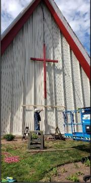
Installation of the cross was quite an undertaking. A bucket truck was rented and the cross was lifted up and installed on the front of the church. You can see George up in the bucket during the painting and the installation.
